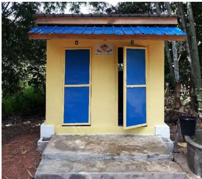
28 toilets were built in 3 village communities
